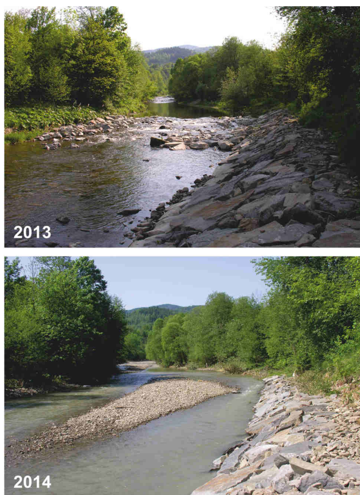
Figure 1. View of Krzczonówka Stream in the vicinity of one of study cross-sections shortly after installation of a boulder ramp (2013) and after the passage of the flood of May 2014. Visible the entrapment of a considerable amount of gravel and burying of the boulder ramp.
