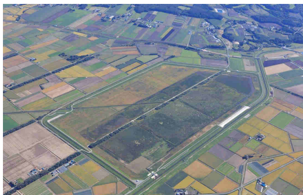
Figure 2 A flood control pond built in the Chitose River, as an example of GI-2
