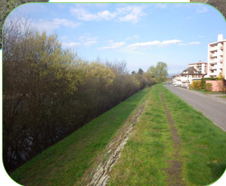
Unmanaged vegetation colonization on dike
