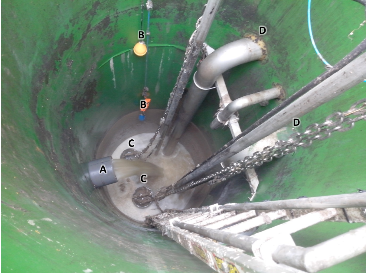
Figure 7: Example of a pumping station. Under A: chamber inlet, under B: water level probes, under C: pumps and under D: pumps exhaust pipes
