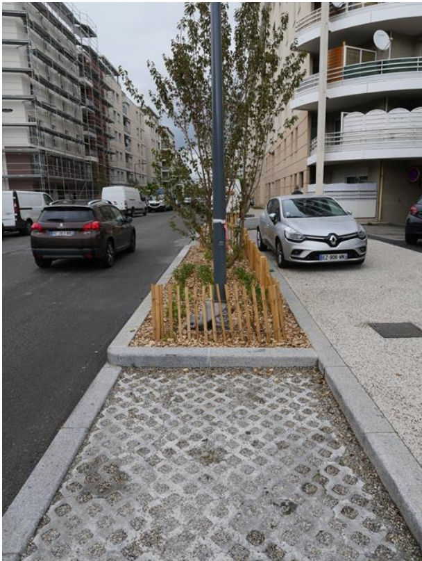
Parking space with alveolar slabs raised over the infiltration trenches.
