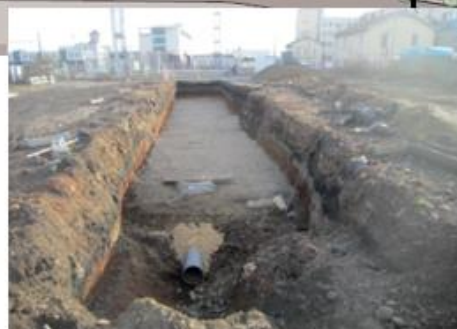
Work on the infiltration trench beneath the prairie
