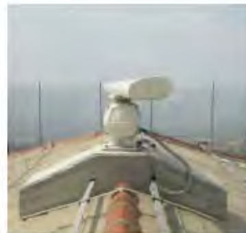
Figure 10: Installation in Genoa, Italy. Please note the clutter net in the background for reducing undesired echoes from waves in the bay and from the city
