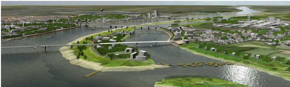
Figure: Artist's impression (left: the River Waal, middle: the island and the new channel, far right: 'De Waalsprong' development)
