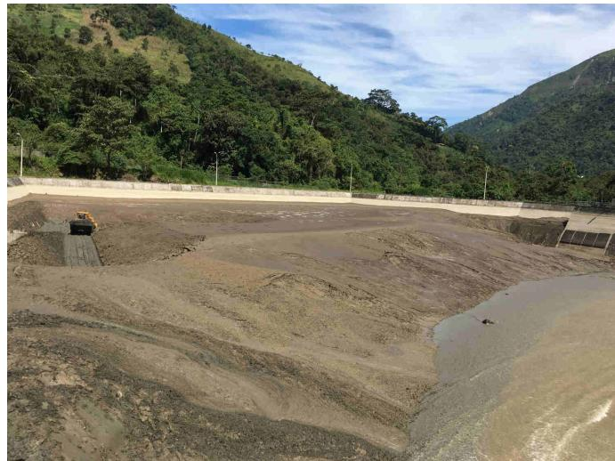
Fig 2. Sediment trapped in the off-stream reservoir of the Ocaña Hydropower Project, Ecuador, during the rainy season Jan - May. (Photos: Tinoco, V.)
