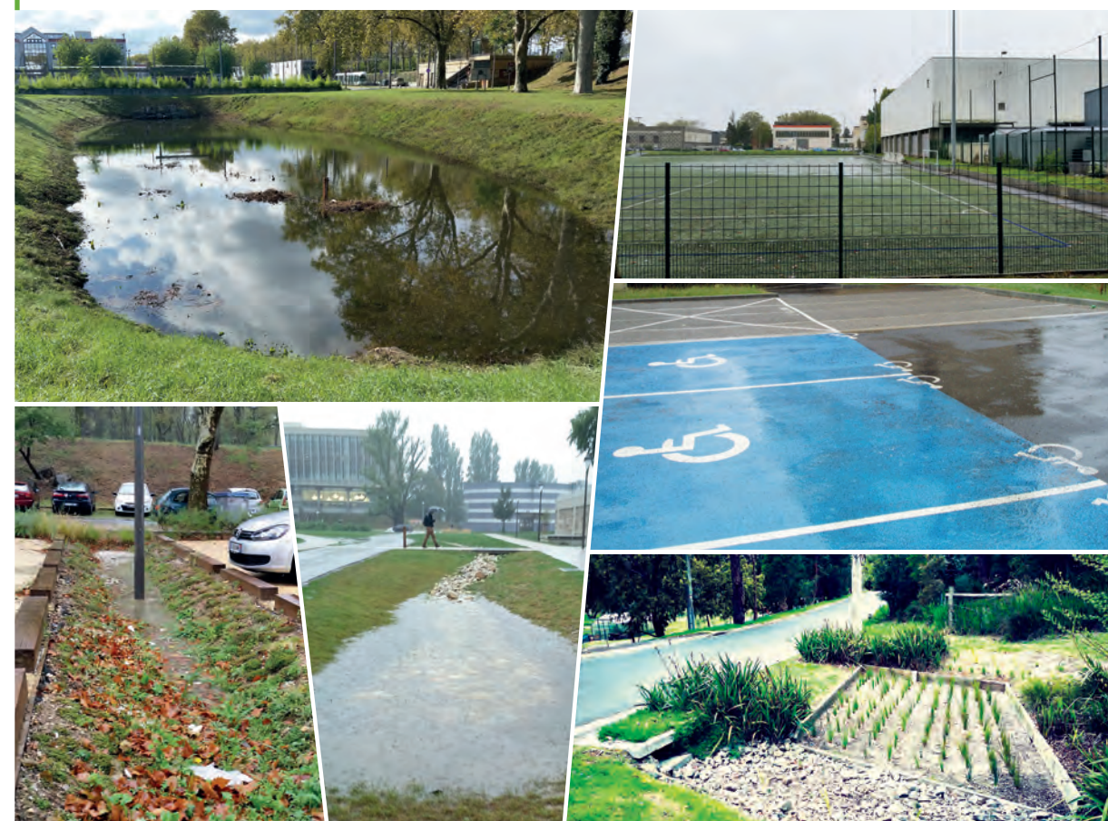
Figure 2: Examples of stormwater management systems: swales, simple infiltration basin, porous and permeable car park, infiltration basin designed as a football playground! (source: F. Cherqui).
