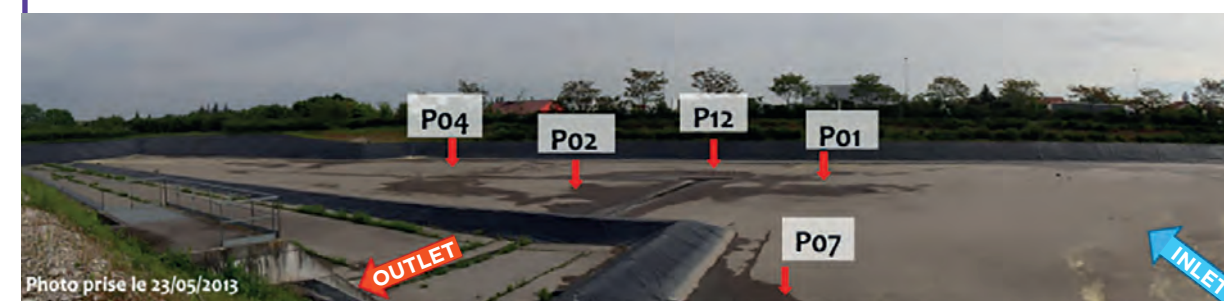
Figure 2: Spatial heterogeneity of organic pollutant concentrations: photo of the Django-Reinhard detention basin and concentrations of Bisphenol A and Diethoxylated Nonylphenol (NP2EO) (P01: inlet, P02: centre, P04: gutter/outlet, P07: outlet, P12: hydrocarbon pit).
