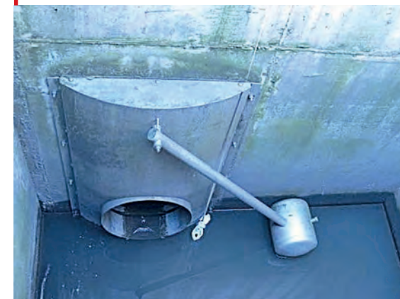
Figure 3: Float valve at the outlet of the Django-Reinhardt detention-settling basin.
