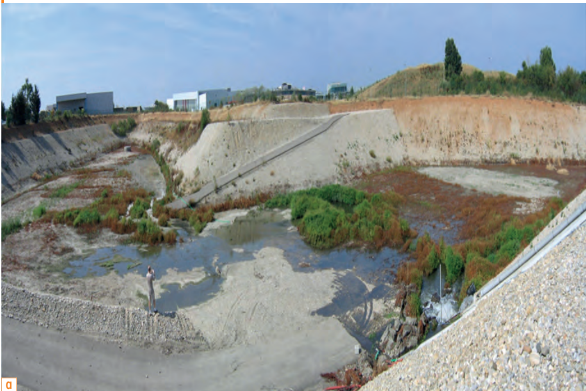
Photos 1: (a) State of the vegetation in the Chassieu-Django-Reinhardt basin between the 2004 clogging (top) and (b) in 2007 (bottom), when clogging began to decrease. (Source : Gonzalez-Merchan, 2012).
