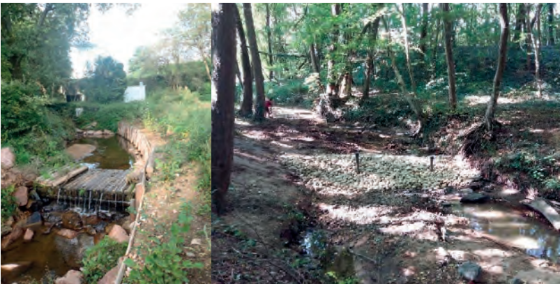
Photo 3: Barrier devices on the Yzeron basin: on the left old (2005) porous weir on the Chaudanne at Grézieux- la-Varenne; and on the right new (2020) porous weir (porous spur) on the le Ratier (source: P. Breil INRAE).
