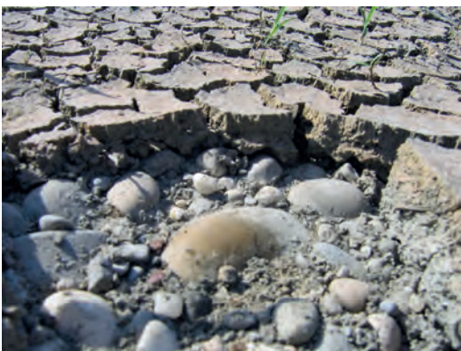
Photo 2: Clogged layer on the Django-Reinhardt basin (source: ENTPE).
