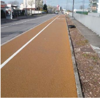
8 km 2 de structures poreuses
